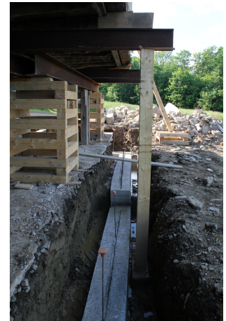
PTF building a frost wall under a raised barn, similar to our foundation project (see their blog for details).
