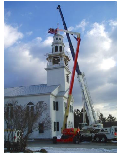
Crane setting up at the Acworth Meetinghouse in 2006 (see http://acworthmeetinghouse.org ).
