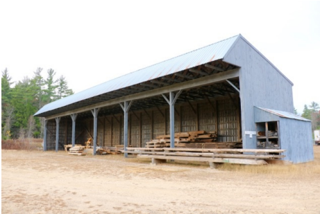
PTF's storage shed and workshop building (lower right) in Nottingham, NH where the tower top, weathervane, and bell will be stored and refurbished.
