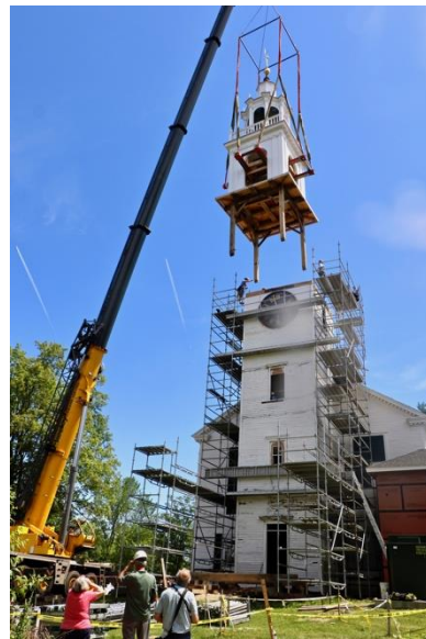
FPCnews-3.jpg — Raising the restored Steeple, June 27, 2019.
