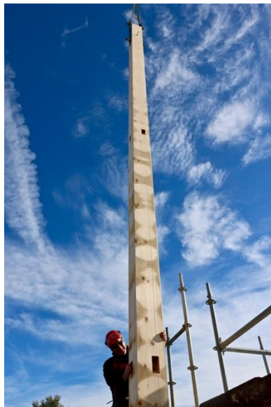
FPCnews-2.jpg — Guiding a 60' tall new corner post down into the Tower as a crane lowers it, Nov. 21, 2017.
