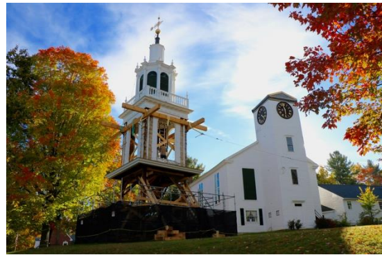
FPCnews-1.jpg — The unsafe Steeple was lowered to the ground Sept. 9, 2015.
